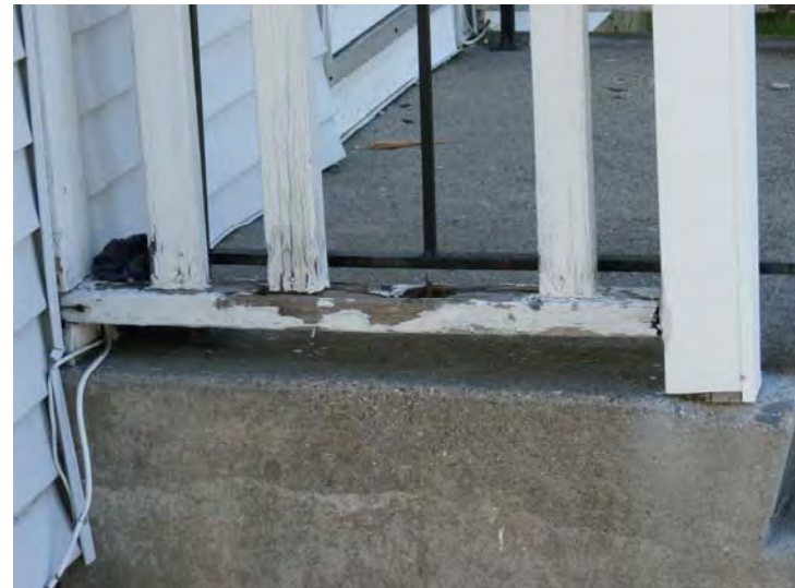
Example of porch deterioration
