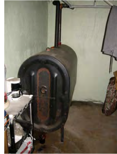
Typical fuel oil storage tank
